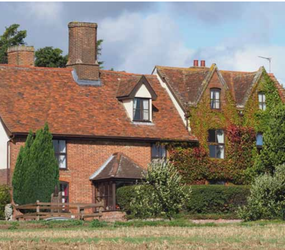
Grade II listed Thornbush Hall
